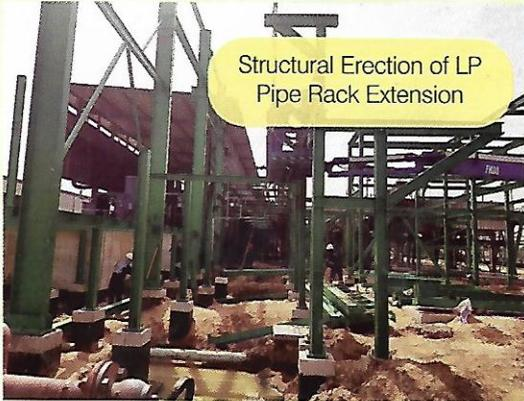
Structural Erection of LP Pipe Rack Extension
