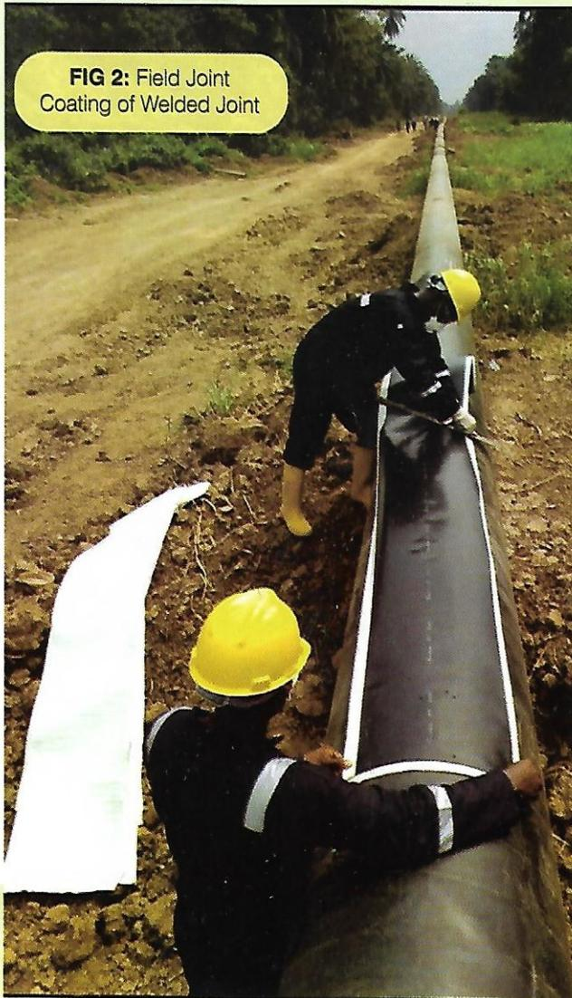
**FIG 2:** Field Joint Coating of Welded Joint
